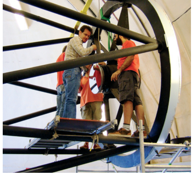
Removing the secondary mirror with the telescope horizontal...
